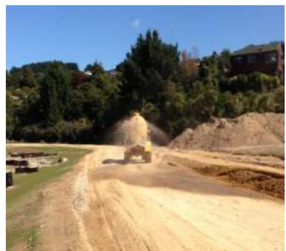
Figure 126: Dust suppression using a water cart
