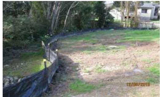
Figure 108: Silt fence
