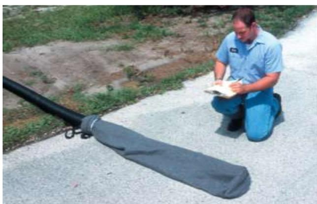
Figure 106: Dewatering bag and pipe sock
