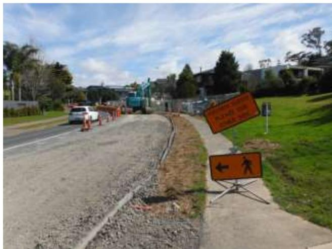
Figure 110: Use of stabilisation products and progressive stabilisation
