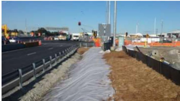
Figure 109: Progressive stabilisation in limited space
