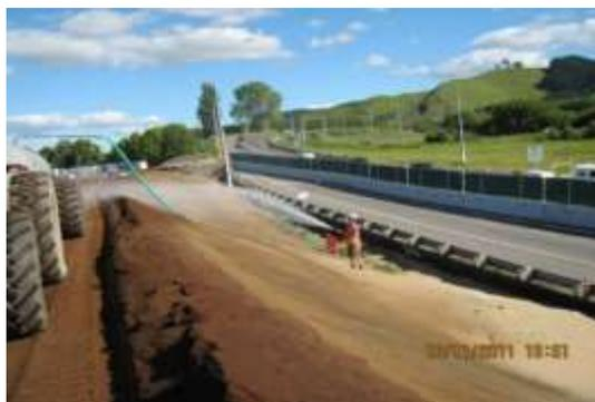
Figure 128: Dust suppression using soil binders/polymers
