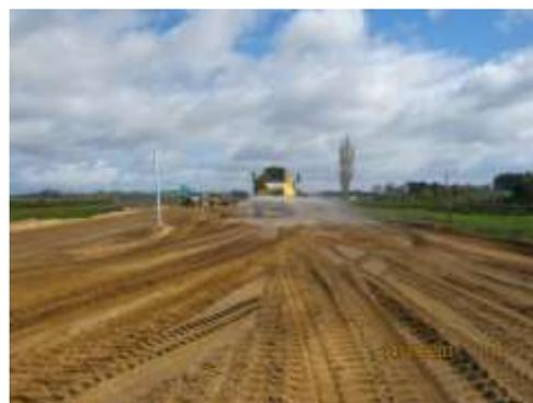
Figure 129: Water truck dampening down the works area
