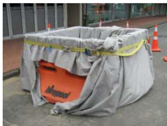
Figure 107: **Example of a mobile 'turkeys nest'** used for dewatering
