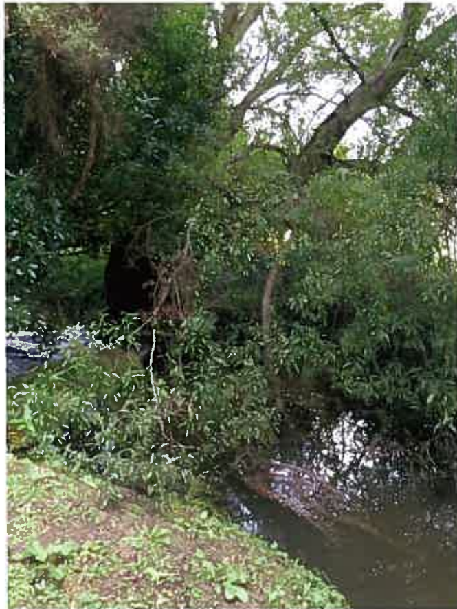
Photo 6 – Willow adjacent to sewer pipe. Note fouling of creek.
