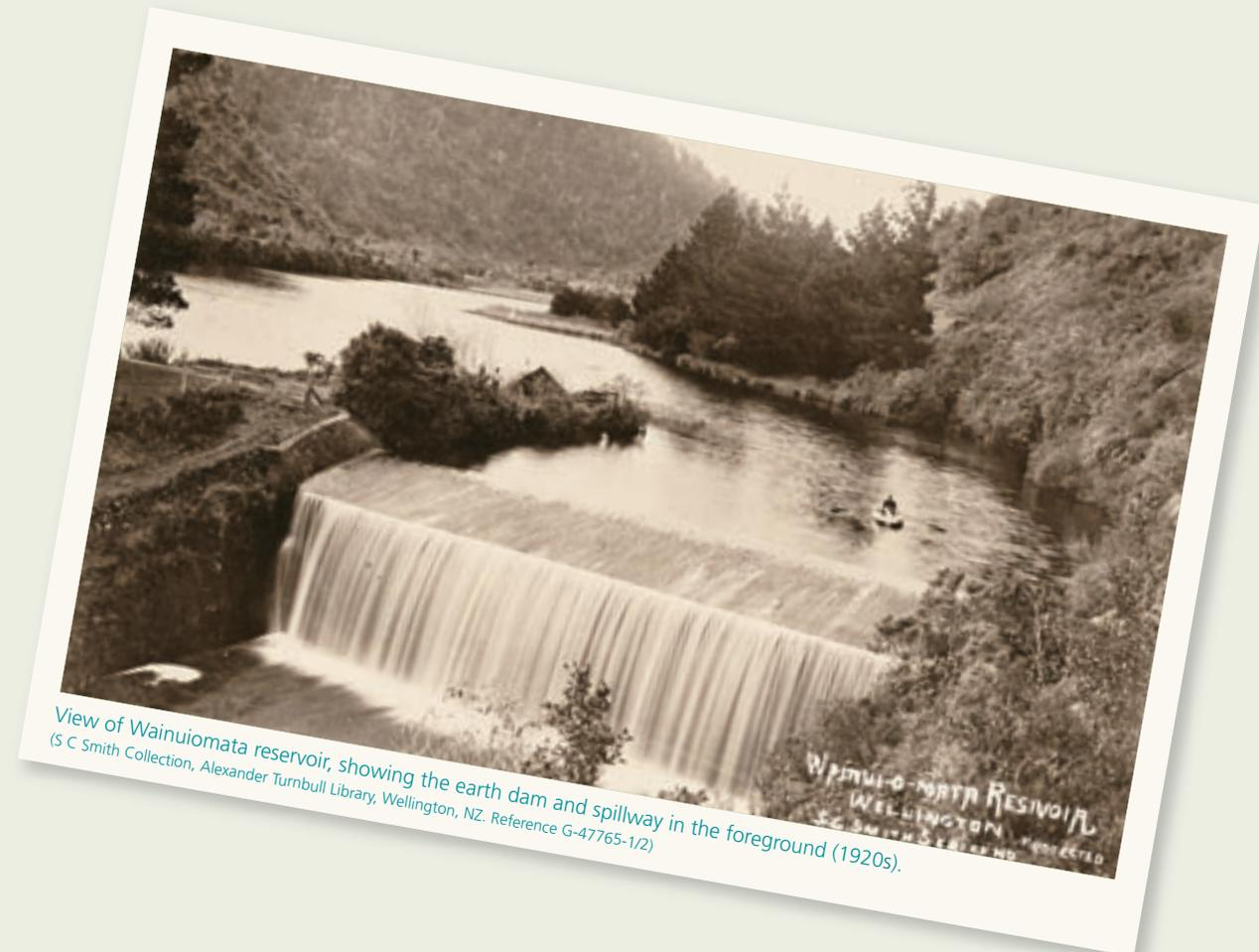
View of Wainuiomata reservoir, showing the earth dam and spillway in the foreground (1920s).
