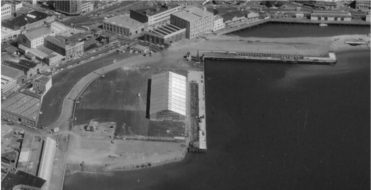
An image of site in March 1969. The breastwork is nearing completion, along with additional reclamation at the bottom of the image. (WA-68374-F, Alexander Turnbull Library)
