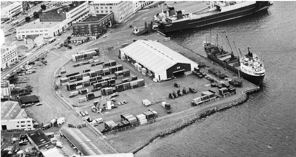
The reclamation and breastwork in 1984. The ro-ro facility was still in use. (EP-1984-5963-F 1953, Alexander Turnbull Library)
