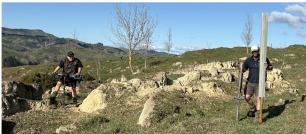
96. Image 16: A brief stop in the work, showing the fractured clay soil of the slip face.
