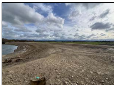
Site 6 - Awaroa Sill, Ruamāhanga Awa - construction still in progress
