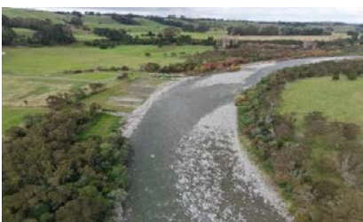
Site 7 – Masterton Raw Water Supply (Waingawa River) – three rock groynes completed.
