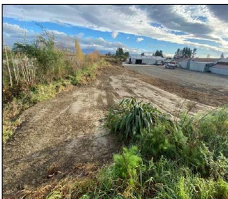
Site 13 – South Masterton Stopbank (Waingawa River) – removal of three trees and the remediation of a section of contaminated stopbank
