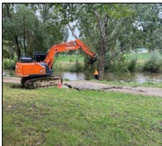
Emergency works in urban reach flood 16th Feb 2026.
