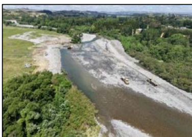
Ruamahanga River - Bed Recontouring works (near Rathkeale College)
