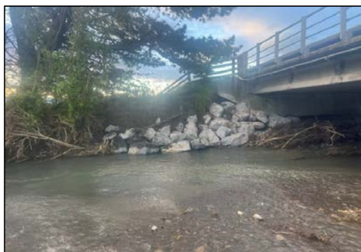
Erosion repairs (rock Protection) to Tauanui River Bridge
