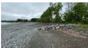
Site 5 – Fullers Bend – seven rock groynes and a 197m rock revetment
