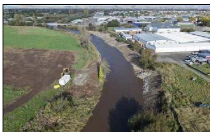
Site 4 – Waipoua Industrial Site (Akura Road) – five rock groynes and a 15m rock revetment completed.
