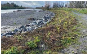
Site 5 – Fullers Bend – offset mitigation planting completed.
