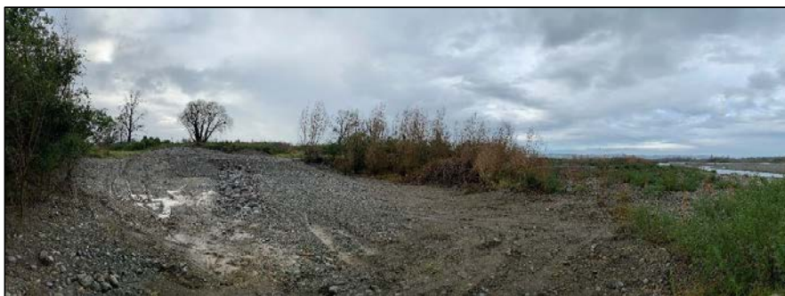
Site 8 – Hood Aerodrome (Waingawa River) – four rock groynes completed
