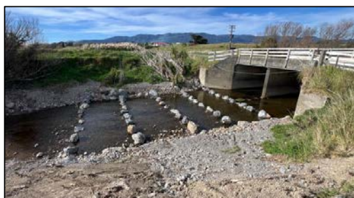
Site 12 – Fish Passage upgrade (Whangaehū Stream/Pā Creek
