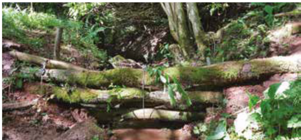
Figure 6: One of a series of woody dams installed in Cumrew beck to reduce flooding in Cumrew Village, near Carlisle, UK. © Eden Rivers Trust
