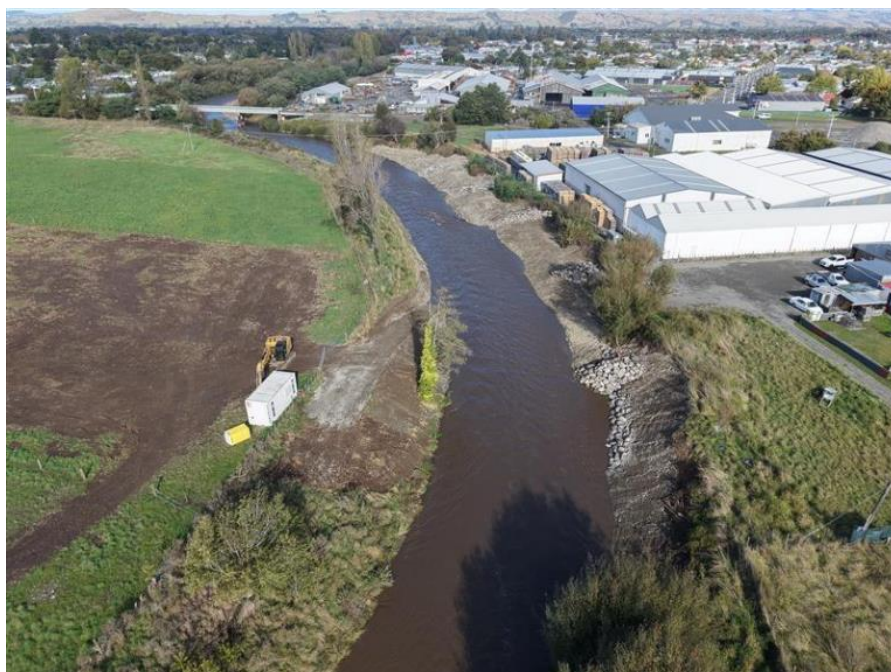
Figure 5: Site 4 – Waipoua Industrial Site (Akura Road) – five rock groynes and a 15m rock revetment completed
