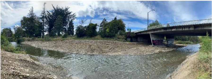
Figure 4: Site 3 – Waipoua SH2 Left Bank – 45m rock revetment completed
