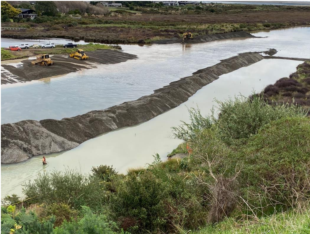
Figure 14: Central channel opened, fish rescue in the true right channel and cross-blading gravel on the true left bank.
