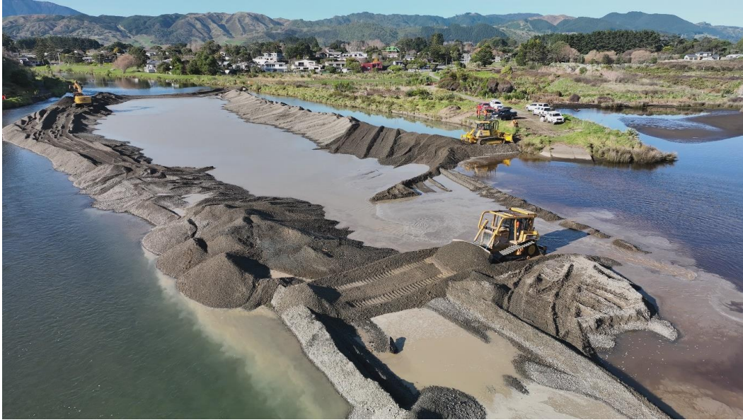
Figure 13: Creating the new central channel through the gravel build up in the Waikanae estuary.
