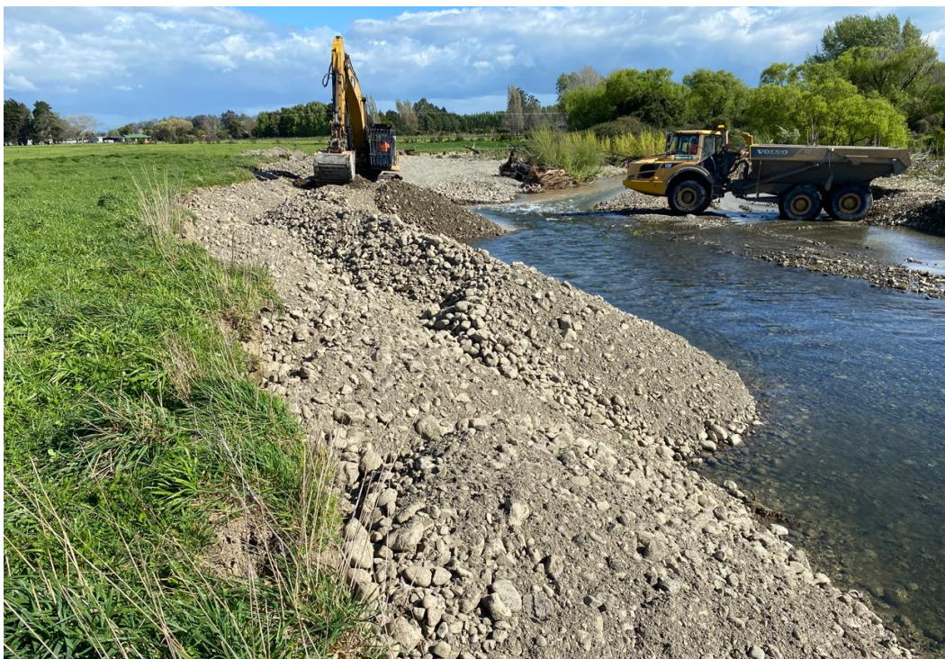
Image 7: Start of gravel infill and bed recontouring.
