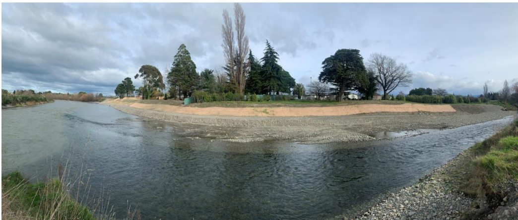
Image 3: Stage 2 (Confluence of the Waipoua and Ruamāhanga Rivers) - Rock groyne and rock revetment completed
