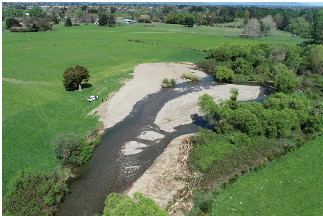
Image 8: Finished works showing infill and new alternate river channel.
