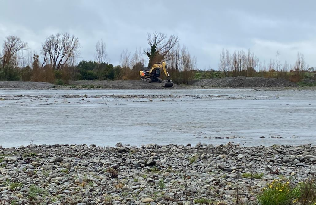
Image 5: Digger shaping up finished gravel groynes
