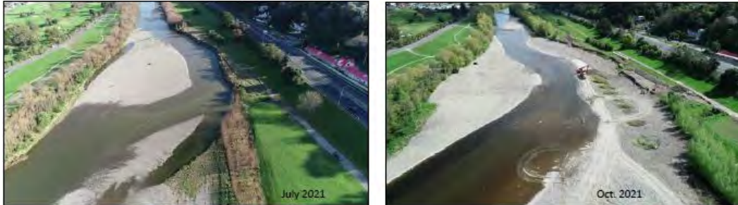
Figure 2. The river meander before and after the lower berm construction.
