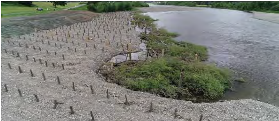
Figure 3. The area complete with willow poles installed.
