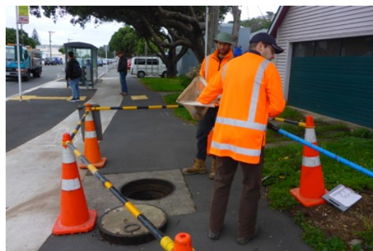
Pae Kawakawa Stream manhole on footpath
