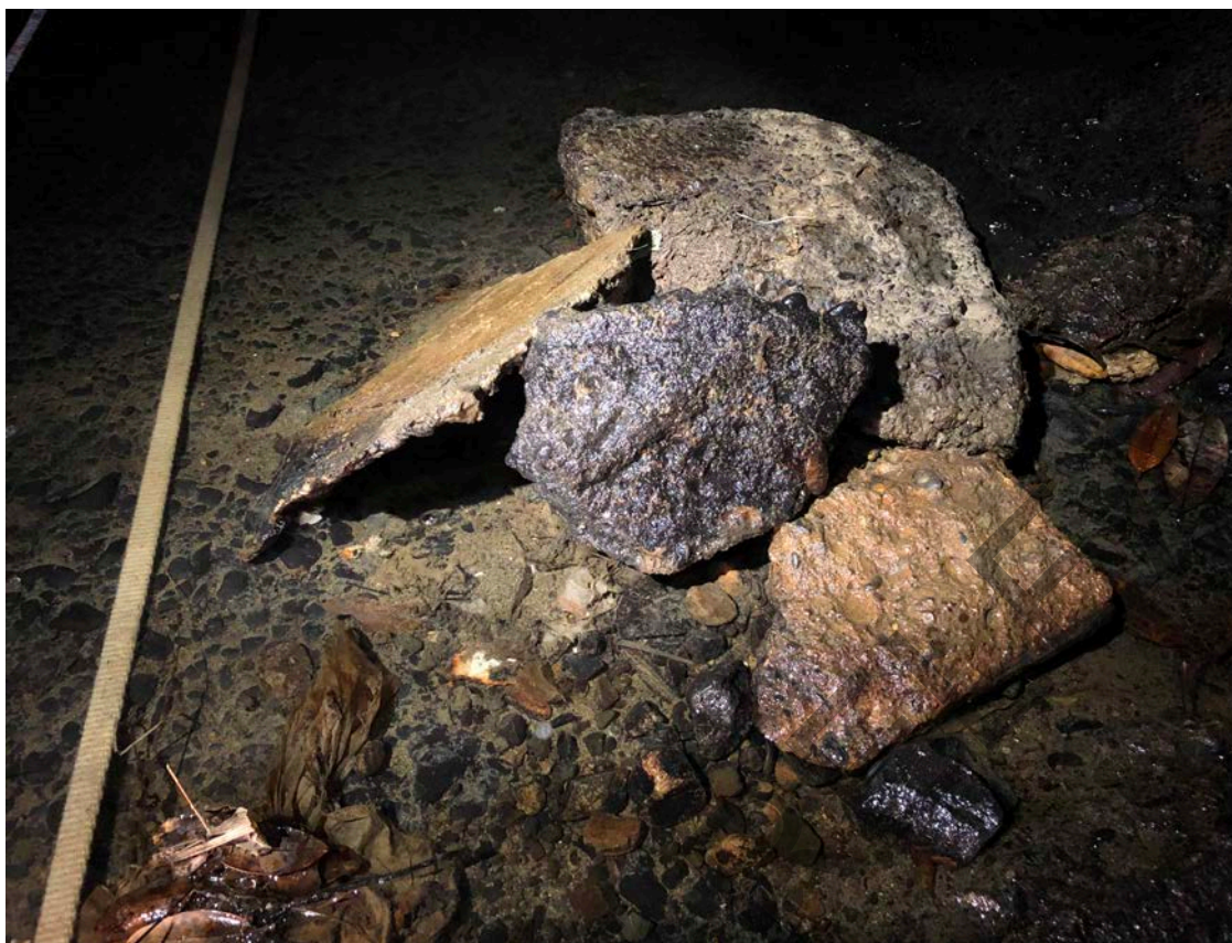
Figure 26 Improvised fish cover feature constructed from rubble found at one piped stream site.
