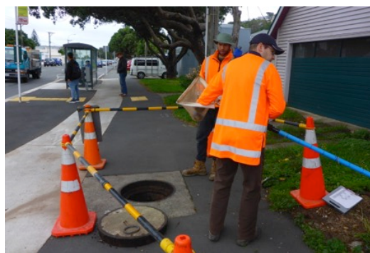
Pae Kawakawa Stream manhole on footpath
