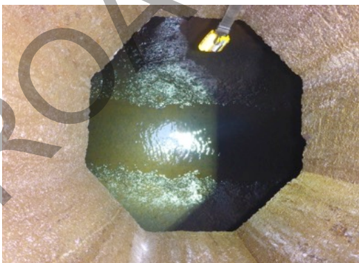
Measuring the atmosphere using a gas detector
