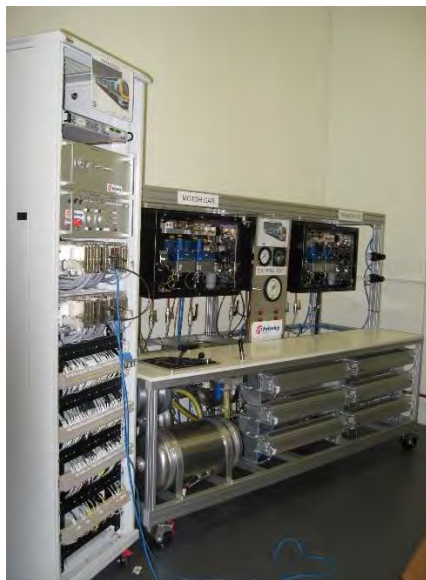
System Integration Test Bench
