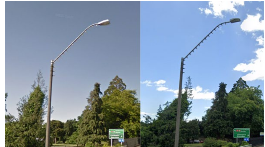
Before and after: Pictured left is the old HPS light and to the right is the new LED light on the SH2 Waipoua River Bridge.
