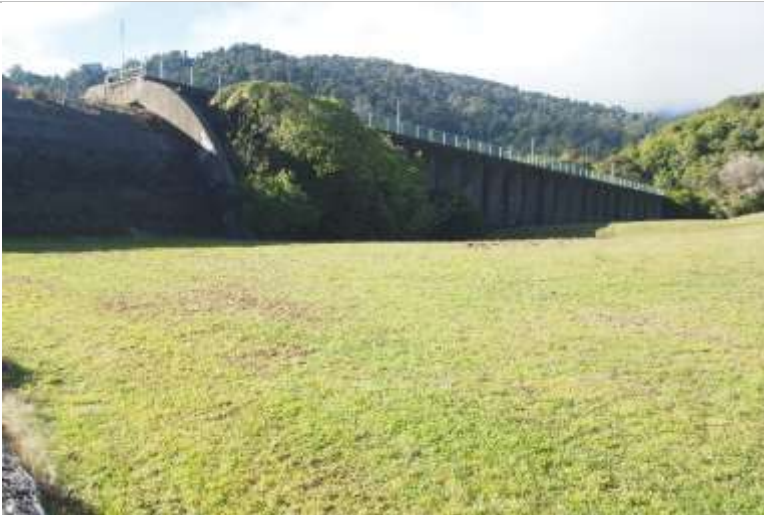
Photo 2: From gate to Wainuiomata River showing dam wall and managed lawn.
