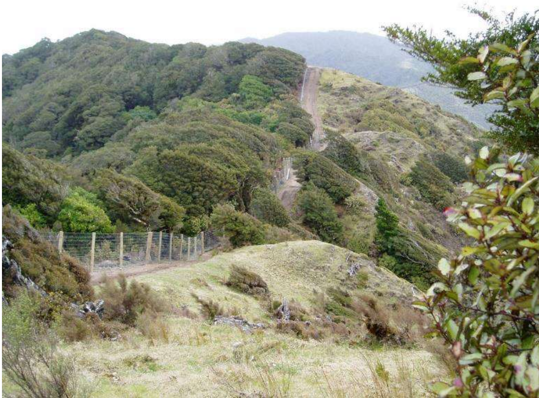
Figure 9. The road and deer fence on the north ridge. Note the hard rock outcrops (see geology below). Photo GW
