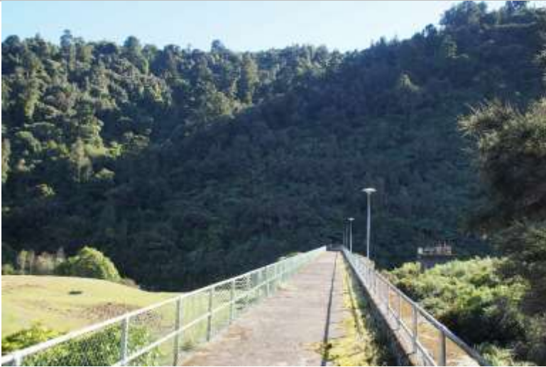
Photo 4: Western Spur from dam wall.
