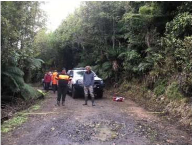
Photo 16: Existing access track at eastern ridgeline. Formed width is 5.9m. Lengths of this track will require widening to provide for both large vehicles and the fence.
