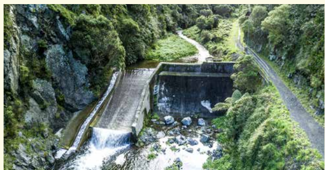
The scenic and historic Woollen Mills dam has been repaired after damage from flooding in May 2015.
