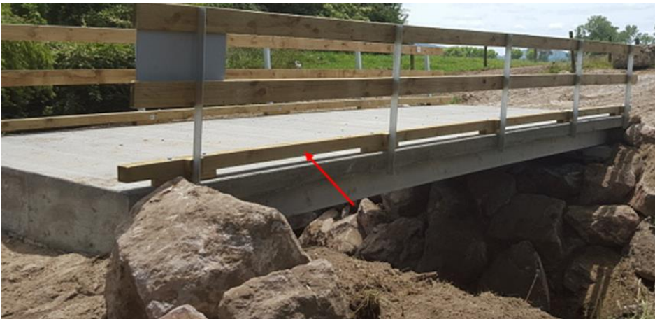
Figure 2-2: Typical rural bridge
