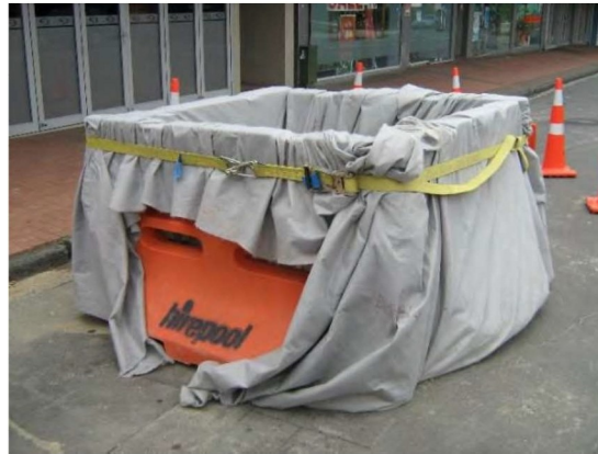
Figure 8.9.2.3: Example of a mobile 'turkeys nest' used for dewatering
