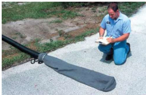
Figure 8.9.2.2: Dewatering bag and pipe sock
