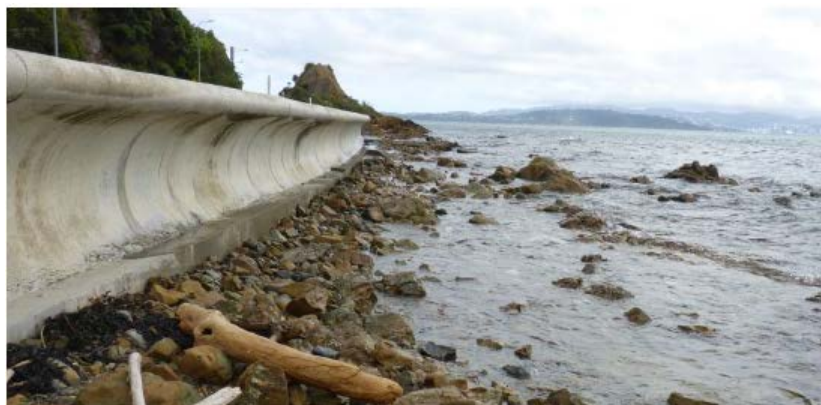
Single curved seawall (York Bay)
