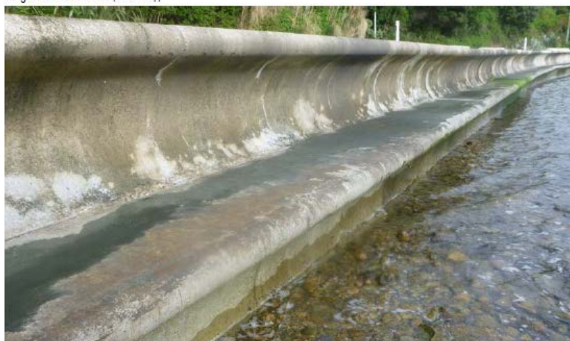
Double curved seawall (York Bay)
