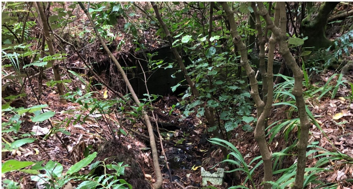
FIGURE THREE: EXISTING INLET STRUCTURE IN INTERMITTENT STREAM
