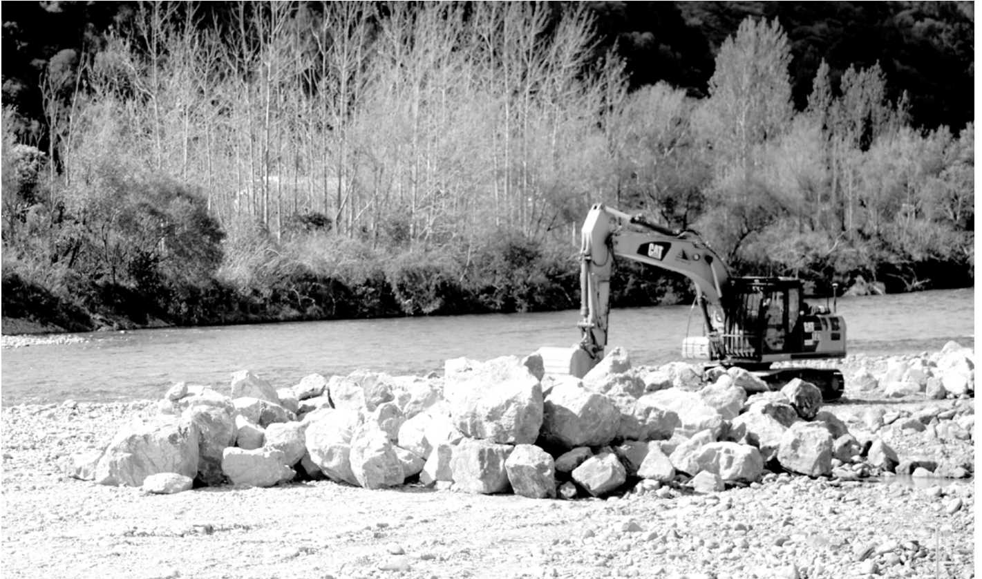
Flood protection work happening on the Hutt River
