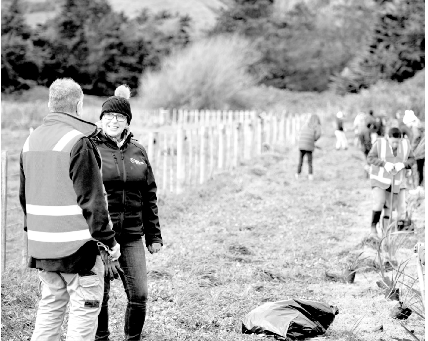
Flood protection work happening on the Hutt River
