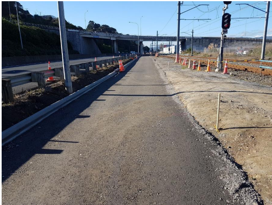
Kerb and Channel – main alignment
