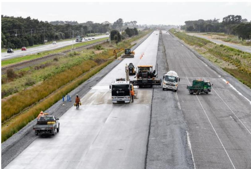
View from Te Horo overbridge – Bridge 8
