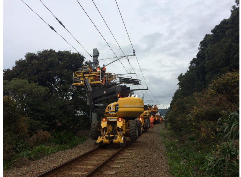
OHLE wiring run at Queens Birthday BOL
