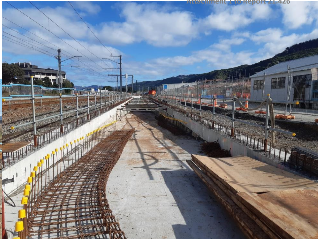
Ramp at Petone underpass taking shape
