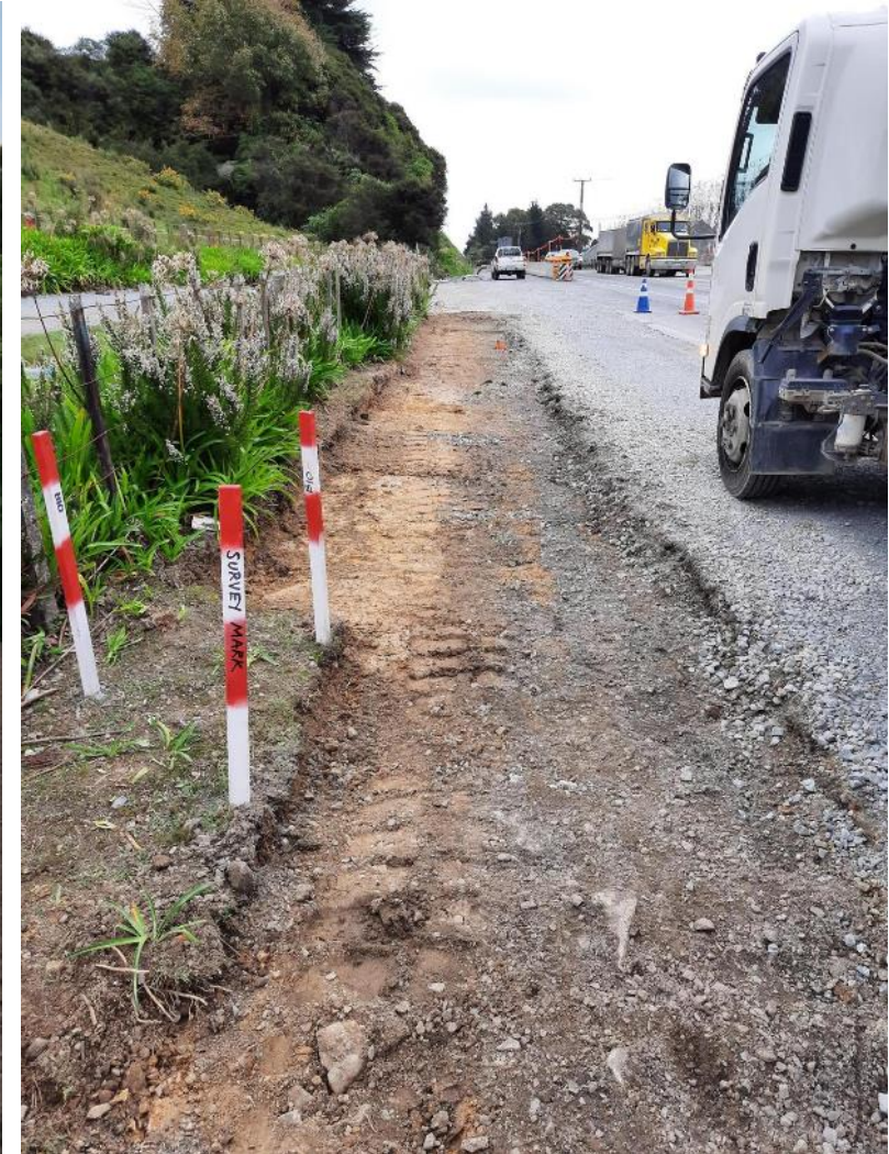
Surfacing preparation works
