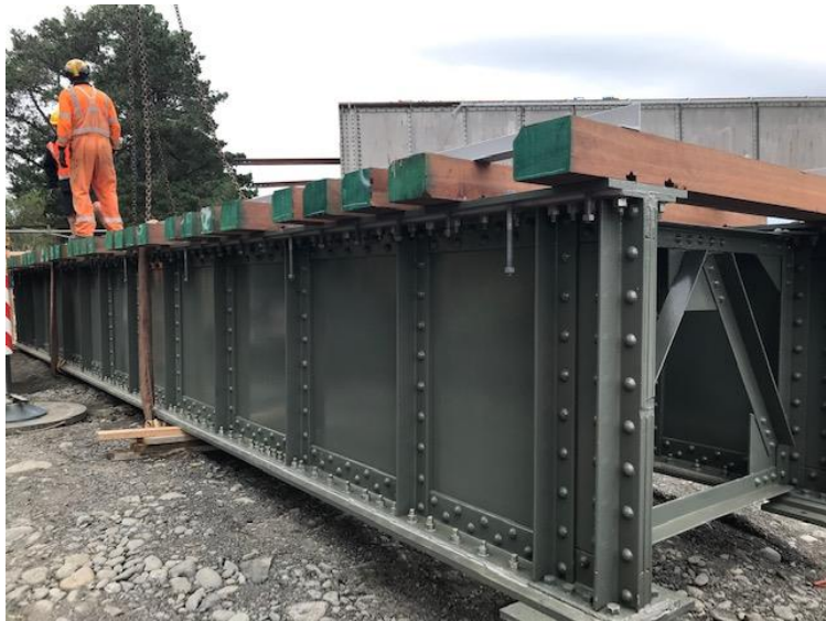
Northern abutment and span renewal on Bridge 49 Wairarapa Line
