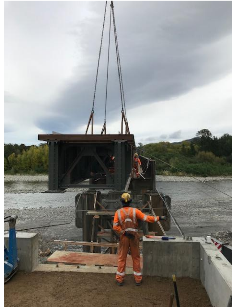
Northern abutment and span renewal on Bridge 49 Wairarapa Line
