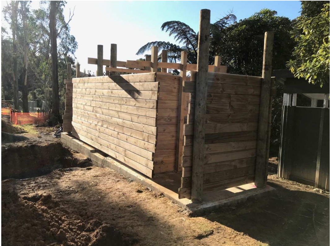
New toilets under construction at Tunnel Gully
