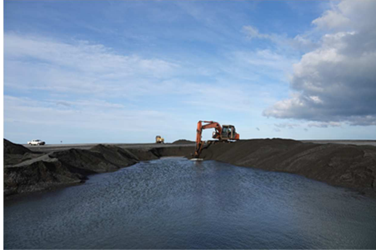
Lake Onoke spit: Mechanical opening to Palliser Bay
