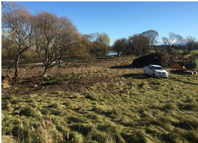
Gladstone River Scheme public area at Wardells Bridge
