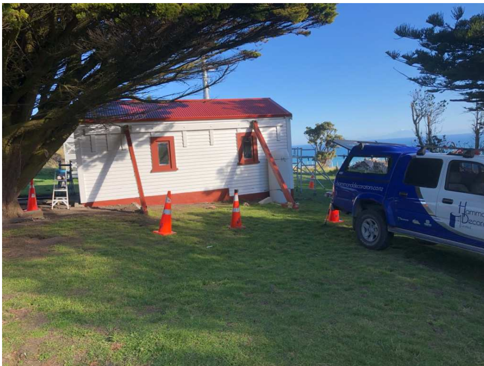
Newly painted generator house and historic garage at Baring Head lighthouse reserve
