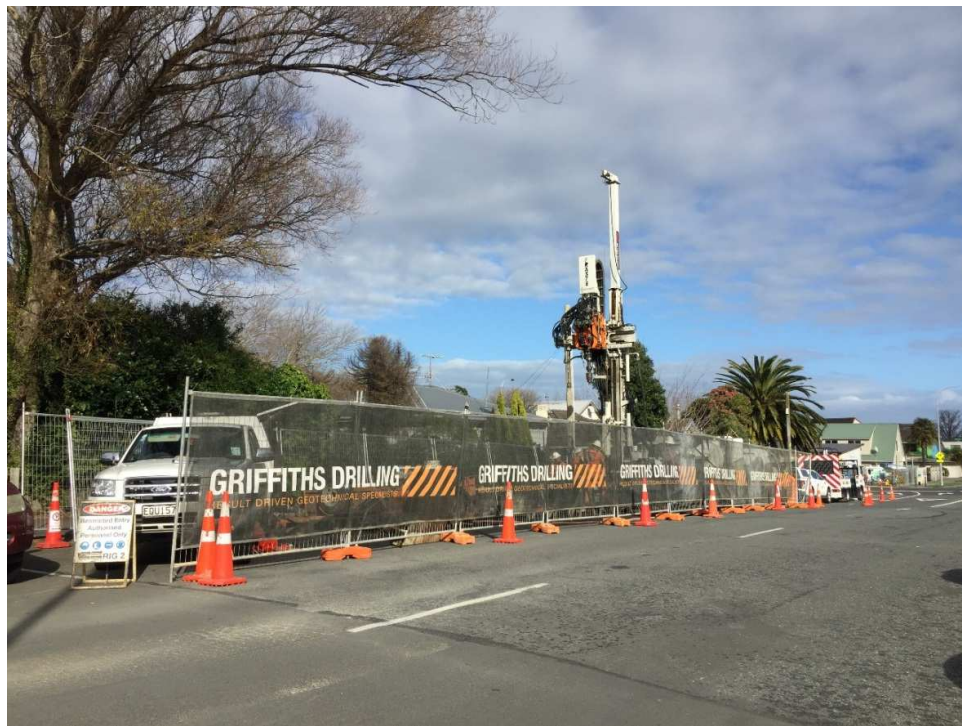
RiverLink Geotechnical Investigations – Griffiths Drilling, Pharazyn St Site, Hutt City
