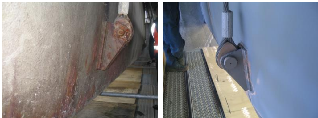
Barrage Gates painting before/after photos – February 2017
