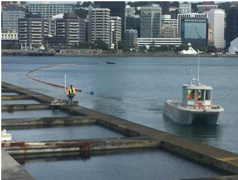
Seacare deploys a floating harbour oil spill boom.
