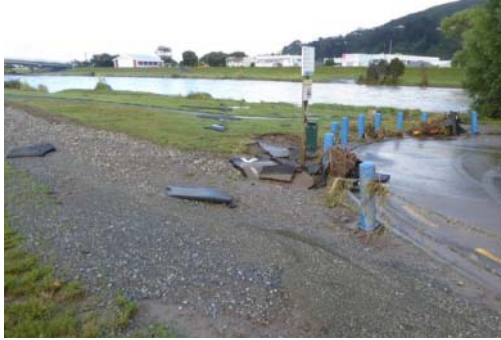
Hutt River car park – asphalt lifted up after flood
