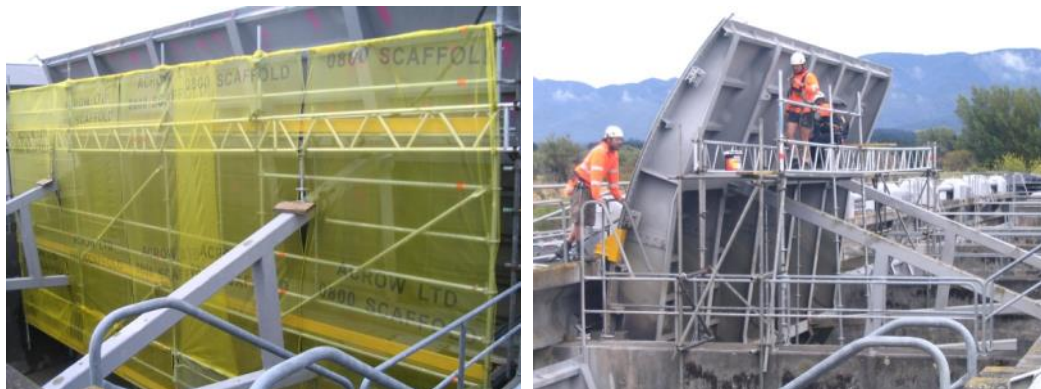
Barrage Gates painting scaffolding – February 2017
