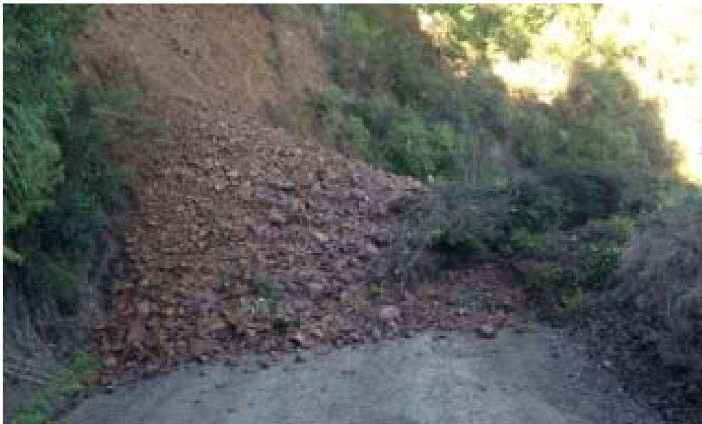
Slip on the Rallywoods Road
