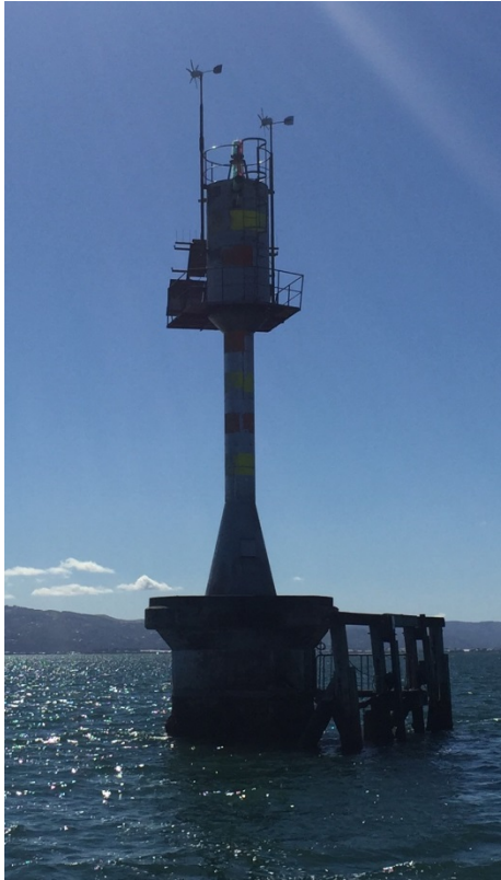
Two wind generators on Rear Leading light structure
