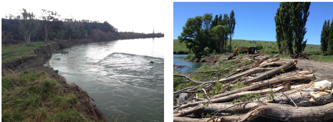
Lower Ruamahanga (Brian Tucker's) bank erosion looking upstream (before) & willow cabling looking downstream (after)
