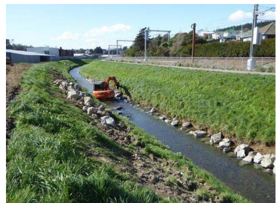
Porirua Stream Wall Place Cut Rock Repairs
