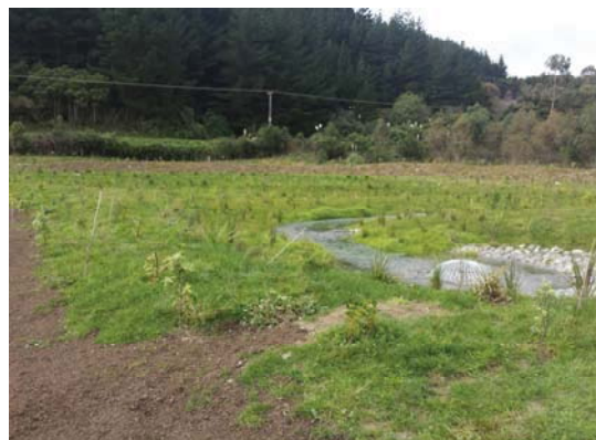
The swale or 'tuna' during the Waikanae WTP opening/powhiri – groundwater being 'naturalised' before discharge into the Waikanae River (via the discharge structure). The groundwater enters the swale at the far end of the channel and flows down the swale to the intake we can see in this photo (where it is then piped a short distance to the discharge structure)
