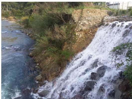
The discharge structure to the Waikanae River – discharging groundwater which has been 'naturalised' through the swale ('tuna') during the Waikanae WTP Opening/powhiri.
