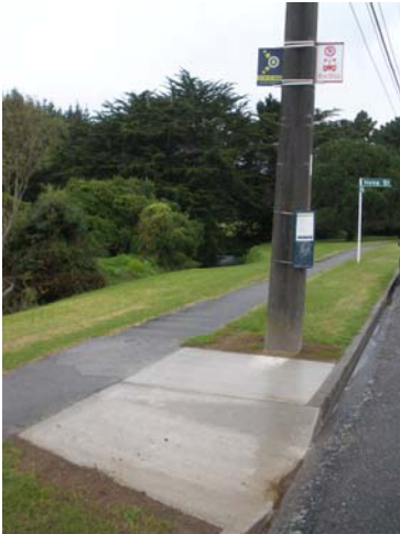
Example of a new concrete standing pad at a bus stop
