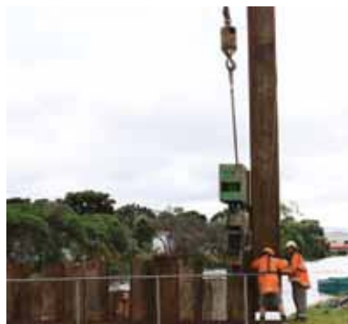
Collecting a sediment sample from the lower reaches of the Waiwhetu Stream for laboratory testing (left) and a pile rig at work installing the first sheet piles near the Bell Road Bridge (right).
