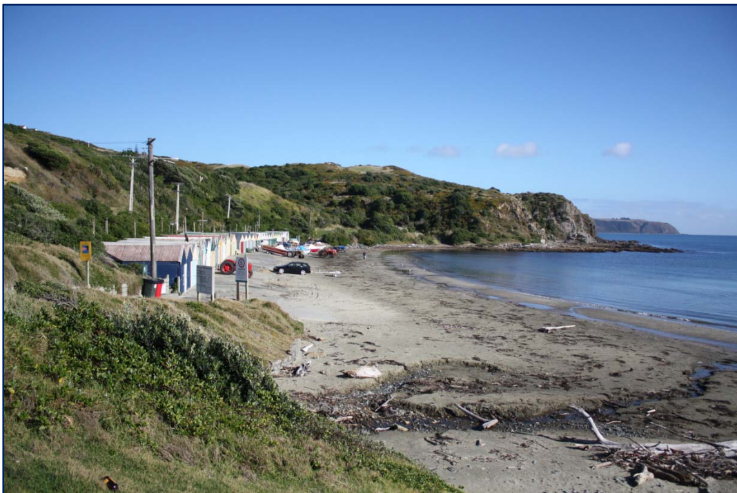
Figure 7: View of the southern end of Titahi Bay beach. Note the impact for the storm water outlet eroding the beach and contributing to the indent in the vegetated dune in the foreground. The vehicle access-way leading to the boat sheds in the centre left will be contributing to loss of sand inland.
