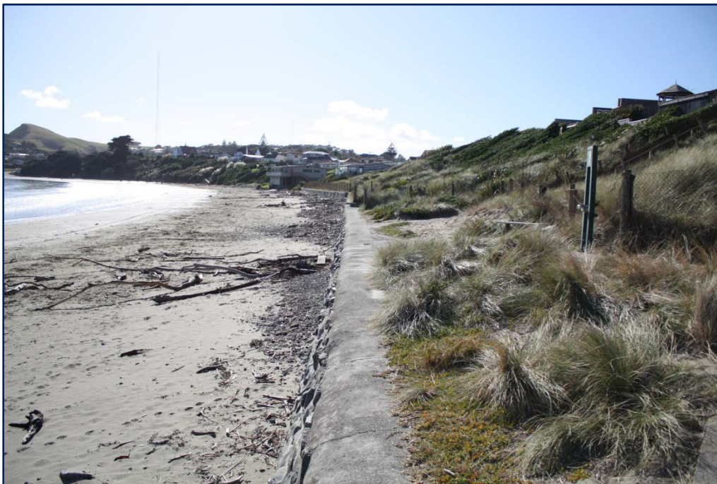
Figure 5: View along the seawall that dominates the central portion of Titahi Bay beach. The seawall is located at or near high water mark where the active foredune zone that historically native sand binding plants is likely to have occurred. Analysis of shoreline positions on aerial photographs since the 1940s indicates the shoreline position has not varied significantly.
