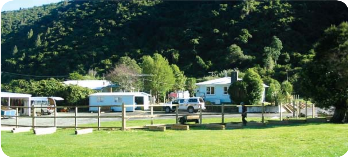
Building a new fence around the Rangers' houses
