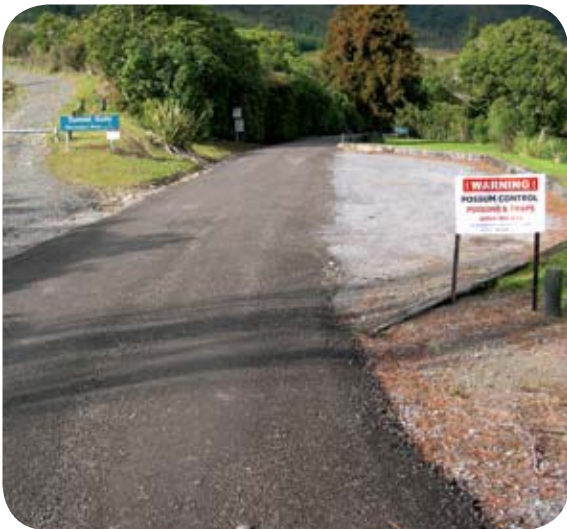
Millings were laid on the Tunnel Gully entrance road to create a hard surface
