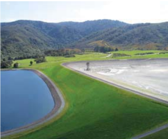
The northern storage lake at Te Marua was empty until late November, to carry out repairs.
