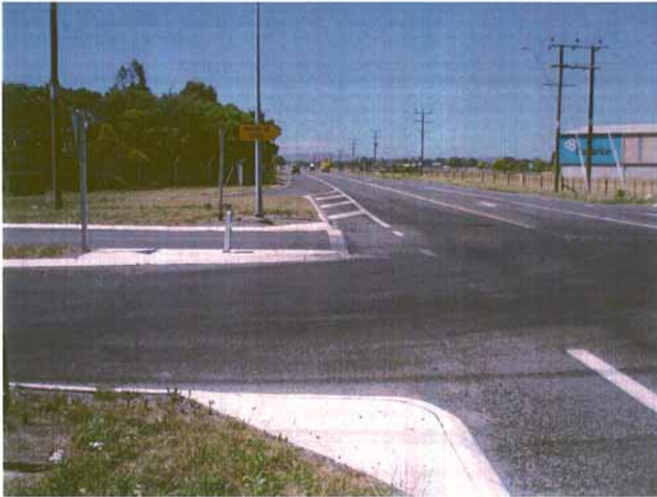
FIGURE 3: Northeast highway approach at Norfolk Road
