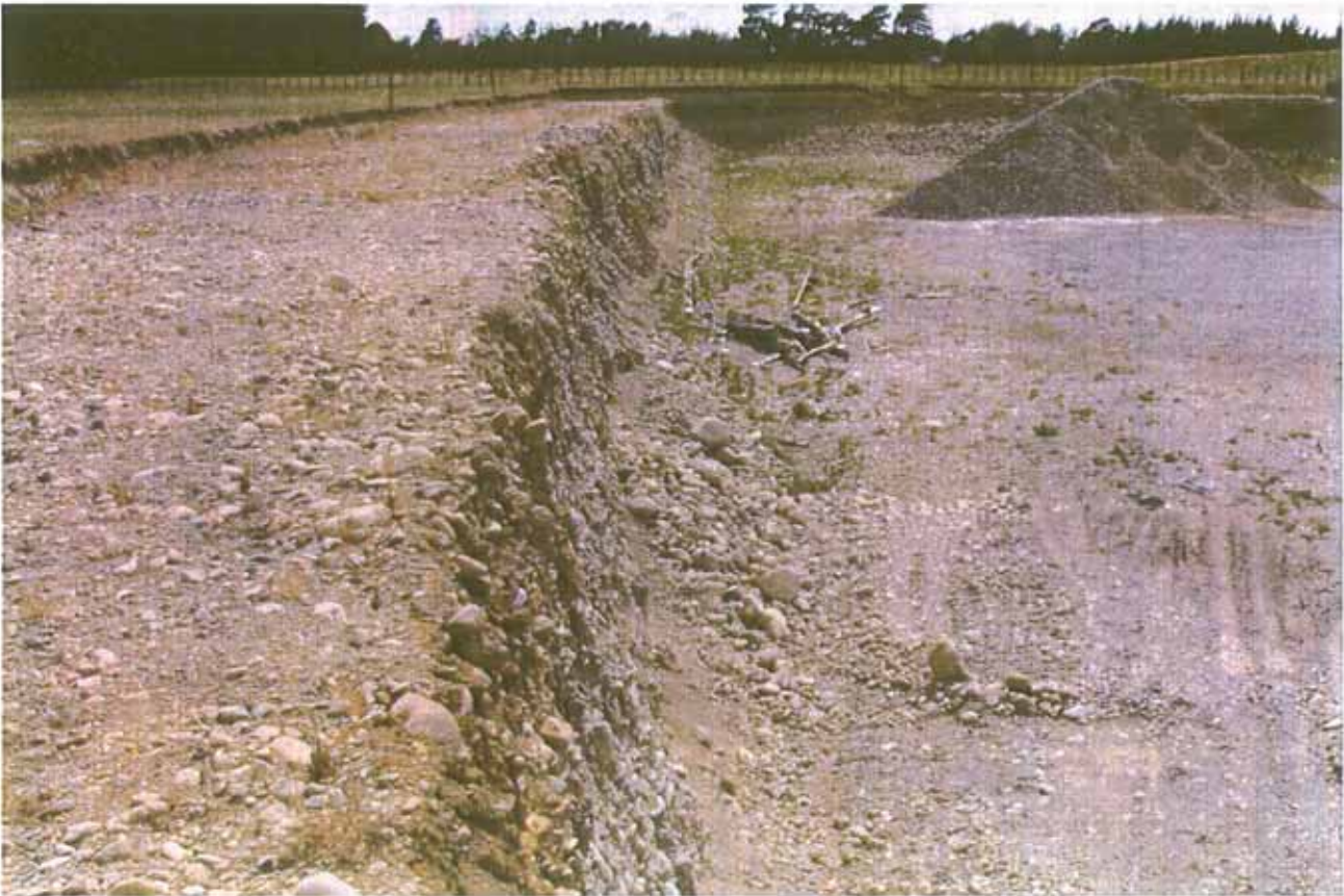
Figure 9. Existing quarry excavation face, up to 4m high. Looking Northeast.
