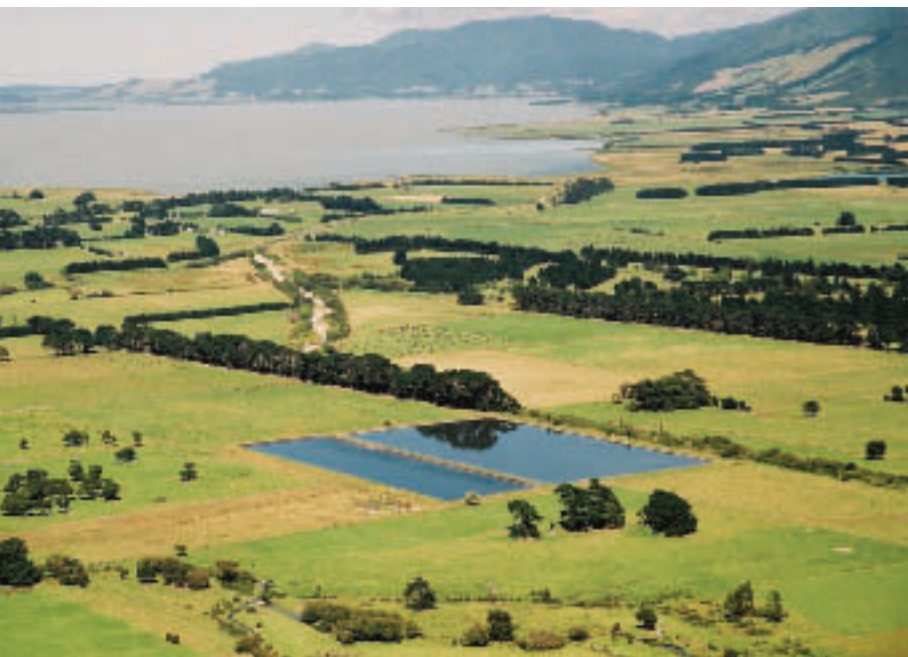
These oxidation ponds, which treat Featherston’s sewage, discharge to fresh water.
