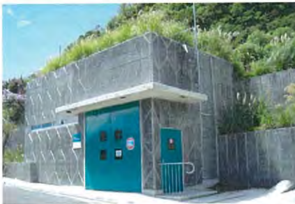
New Karori pumping station with its green roof
