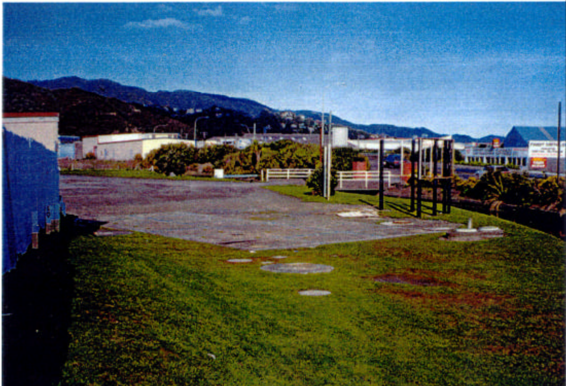
Figure 2 Existing Valve Chamber located under carpark at Randwick (above ground control room on the left)
