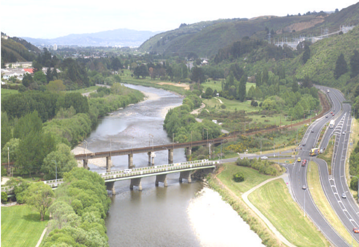
Figure 2 : Silverstream Bridge – water main located on upstream side of the Bridge
