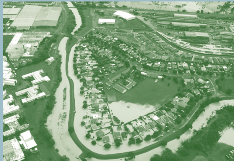
Flooding at Riverside Drive from the Waiwhetu Stream, 15-16 February 2004
