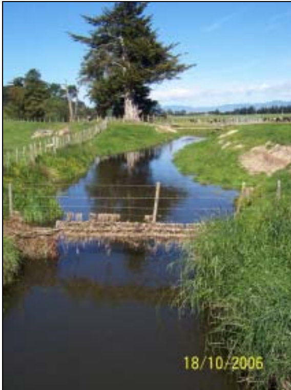
Figure 8: Otukura Stream looking downstream from Wards Line
