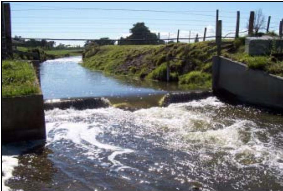
Figure 13: Greater Wellington flow monitoring station Otukura Stream at Weir
