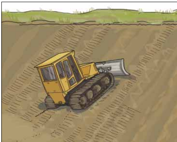
Excavator tracks can effectively compact slopes.
