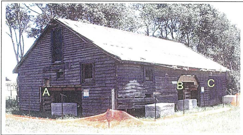
Figure 6. View of barn from north east corner. A = opening cut for removal trailer. B = barn doorway. C = barn doorway with door.
