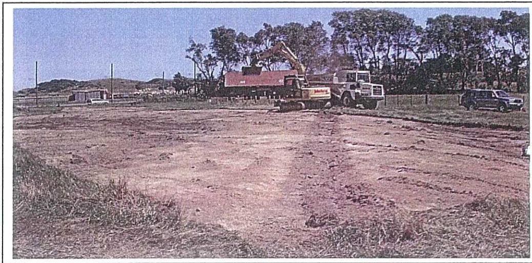
Figure 45. Camp Russell looking southwest showing road and trench with water pipe.
