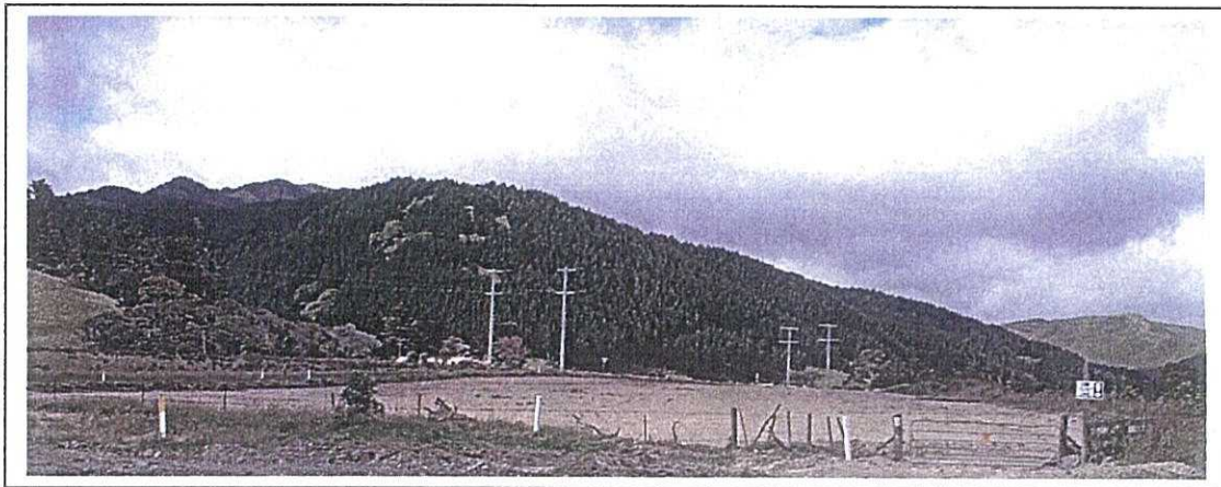
Figure 34. Photograph looking south showing area of topsoil stripping (= A, Figure 33).
