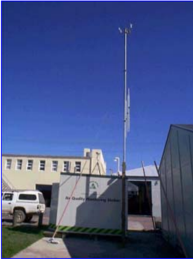
Figure 3.2: Birch Lane air quality monitoring station
