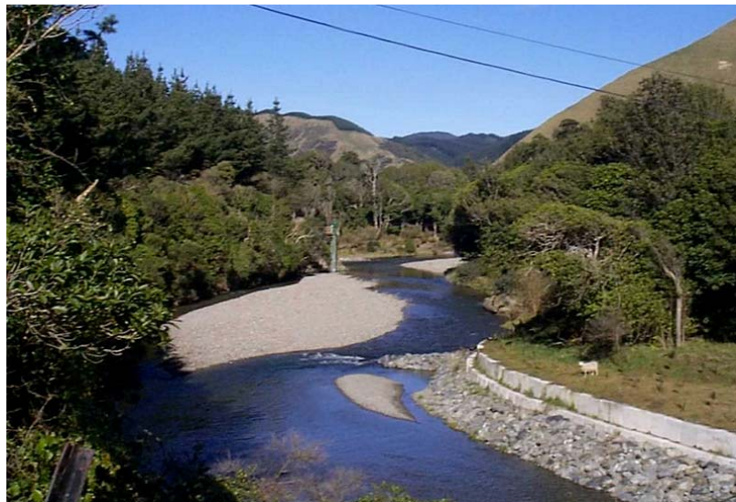
Figure 3: Looking upstream to the Water Treatment Plant reach
